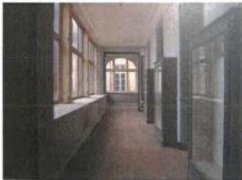
Photo situation 2006 ; couloir (photo P. Sosnowska)
