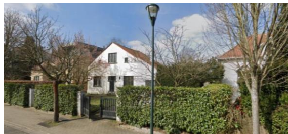
Situation existante © Google street view
